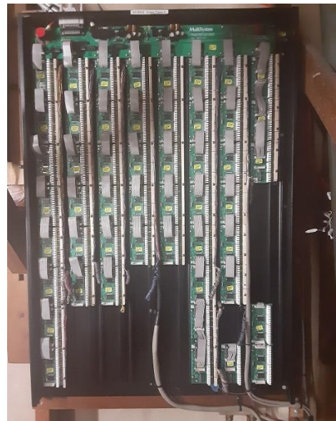
Single board replacing the antiquated four previous boards
